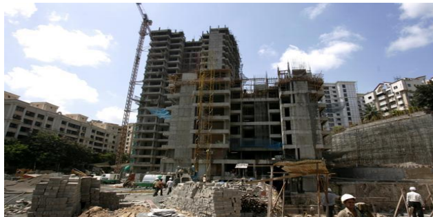
Fig:3.5: Flyash used in construction
